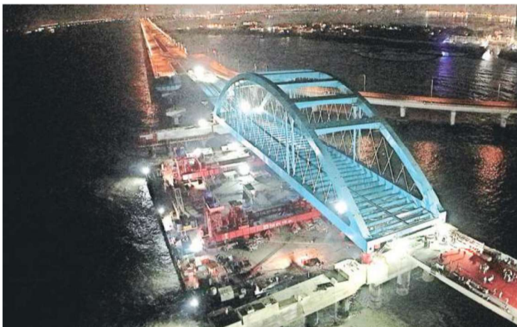
Weighing up to 2,000 MT, the girder was manufactured in Haryana. Express
