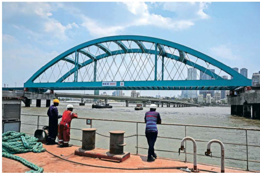
This is the first time a girder was launched in open sea for an infrastructure project in the country. Sankhadeep Banerjee
